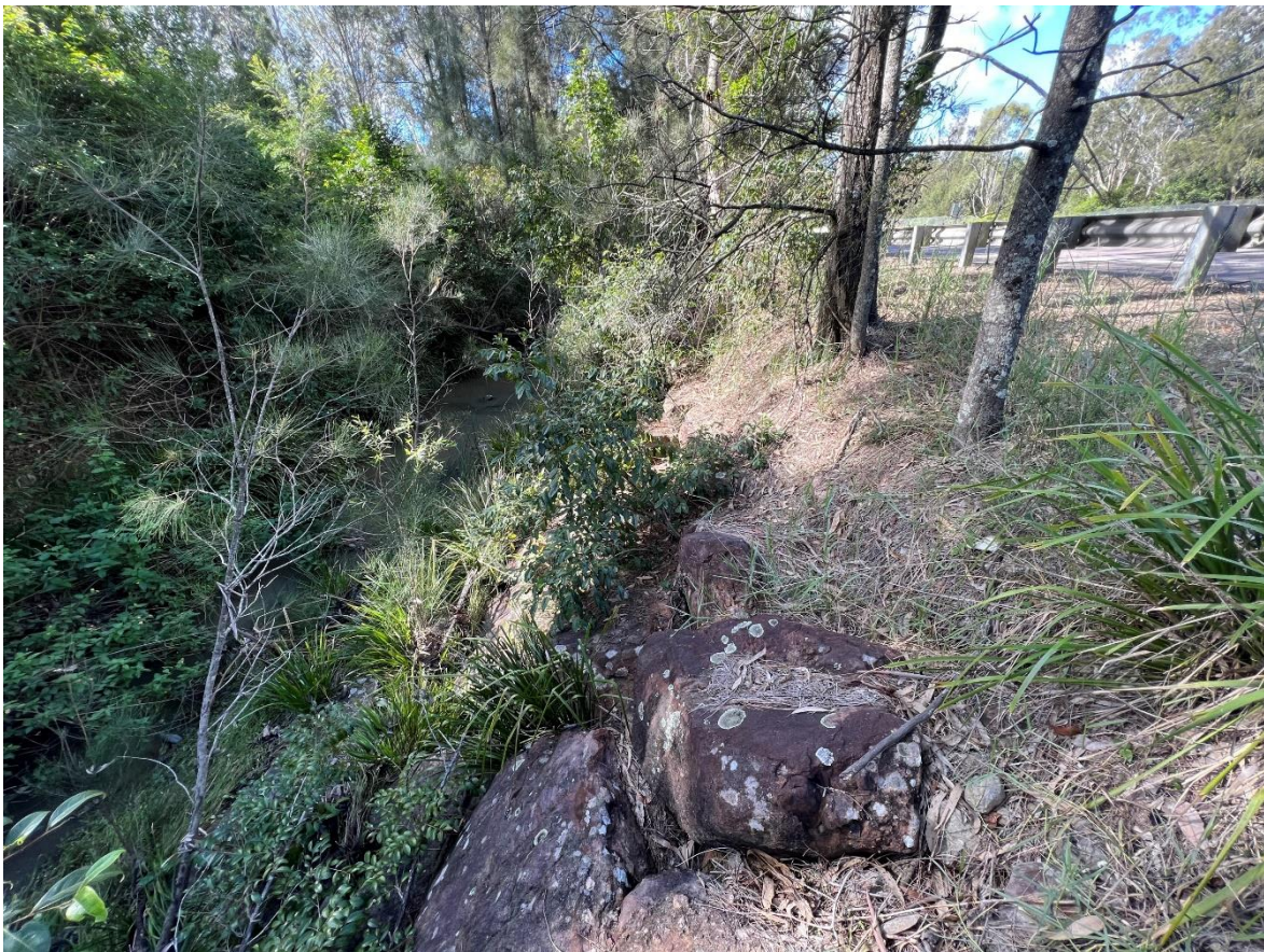
Figure 3.6 Typical northbound embankment, sandstone block wall and chainage channel
