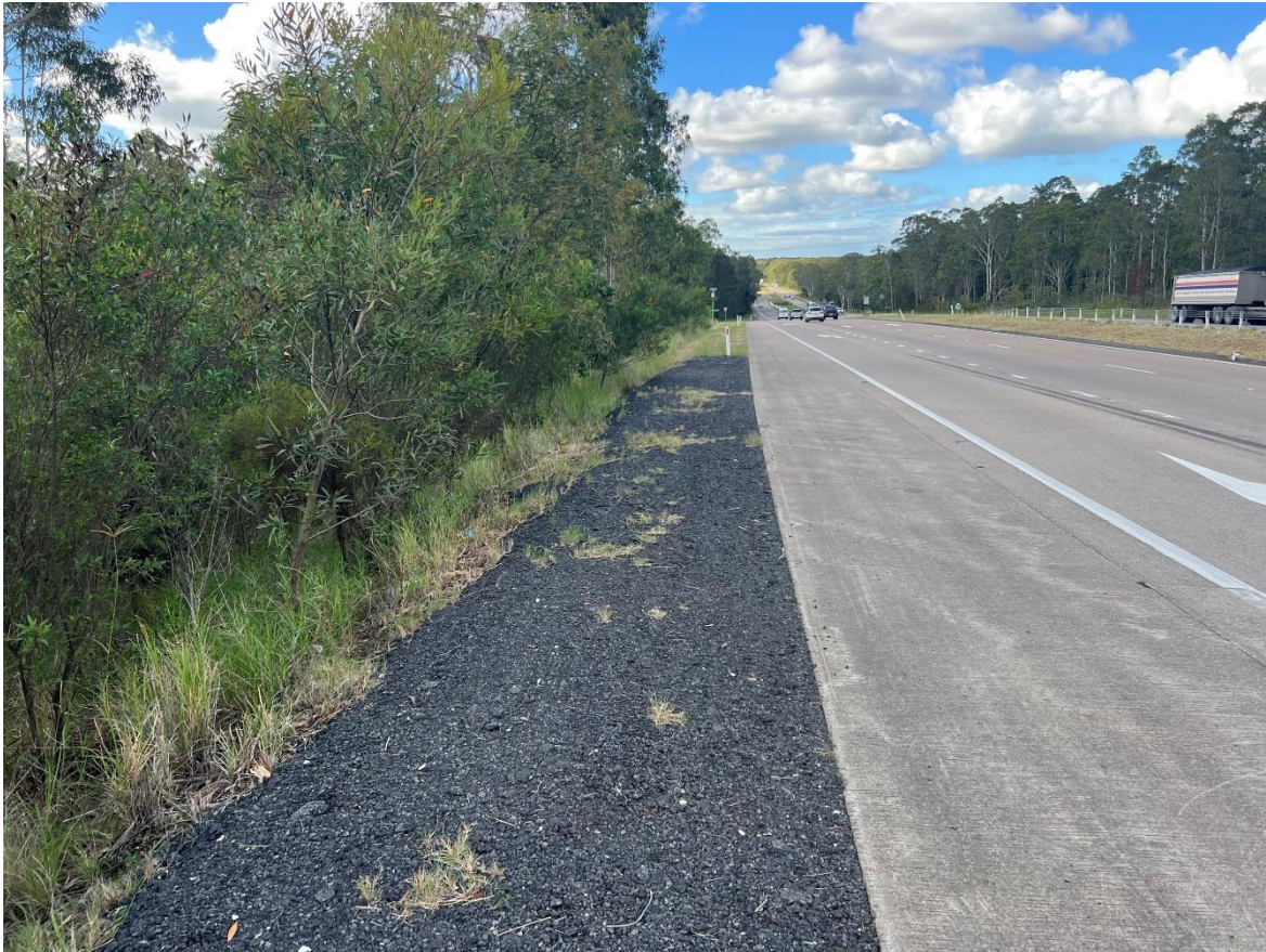
Figure 3.3 Looking north-east along the Pacific Highway towards the intersection
