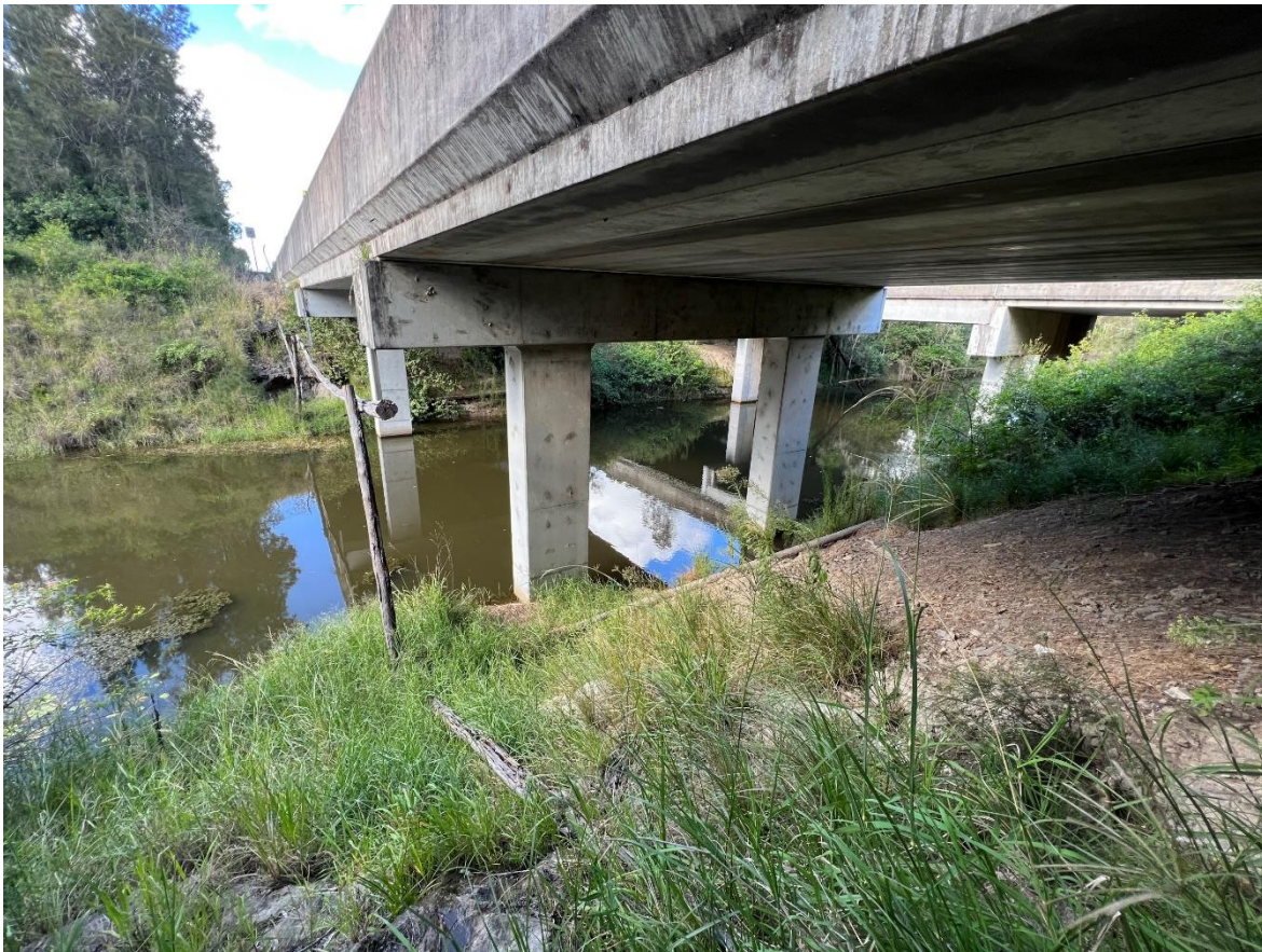
Figure 3.4 Bridge substructure crossing Balickera Channel, looking north-east
