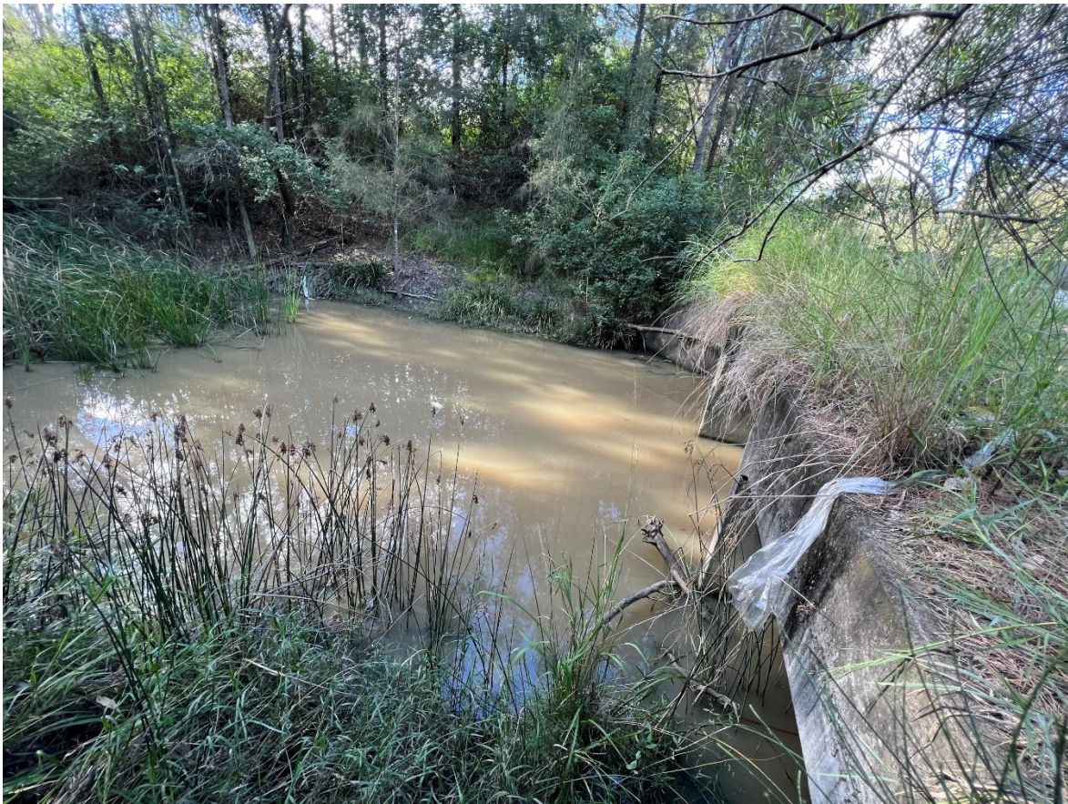
Figure 3.5 Looking north-east to the three-cell box culvert and ponded water
